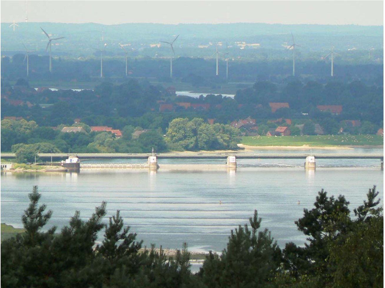
Elbe, Tidewehr in Geesthacht
